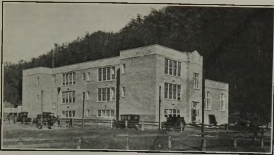
School Building at Caretta, McDowell County, W. Va.
