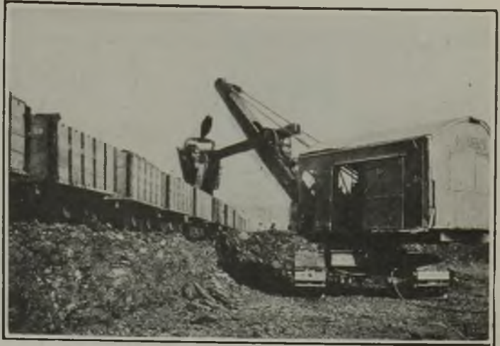
Loading Out Stripped Coal by Power
