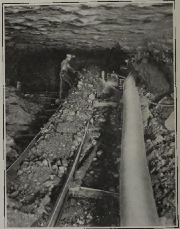
Fig. 2—Looking Along Conveyorway Toward Fan
