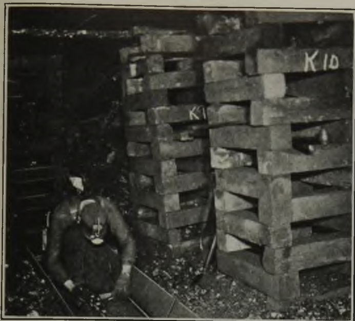
Fig. 8—Shortening Sectional Conveyor
