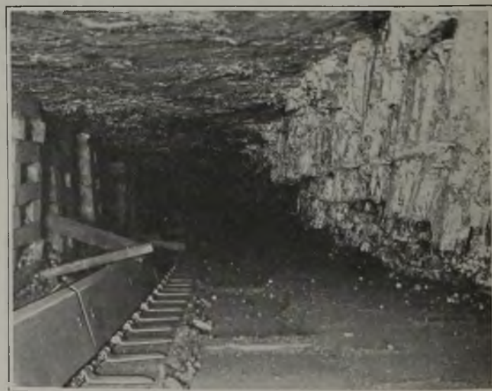
Fig. 2—Long Face After Face Has Been Snubbed
