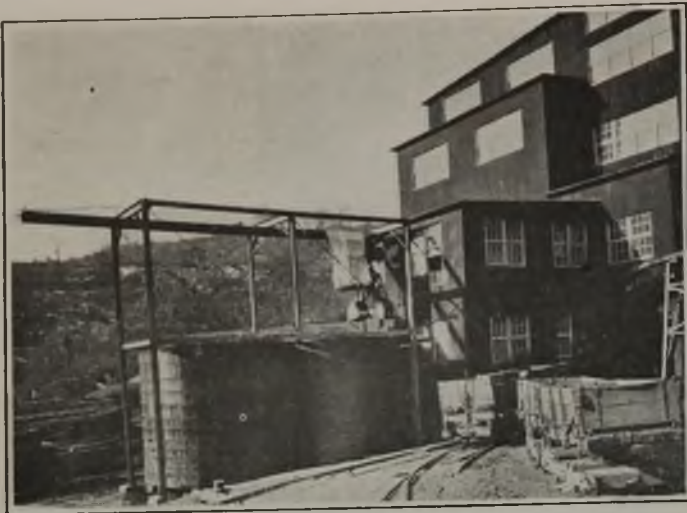
Part of Silt-Recovery Plant at St. Clair
