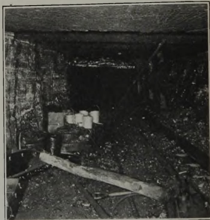
Fig. 7—Sectional Conveyor Into Which Coal Is Discharged by Face Conveyor
