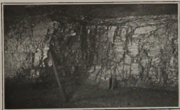
Fig. 8—Face Properly Prepared for a Butt Shot
