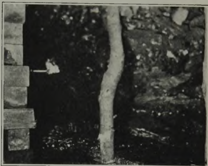
Fig. 9—Safety Prop After Removal of Cribs
