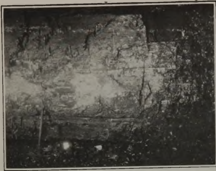
Fig. 4—A Shot Productive of Large Lumpy Coal
