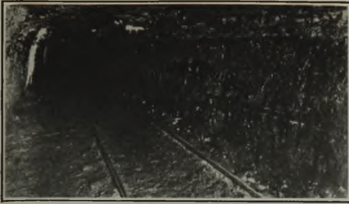
Before Rock-Dusting, Main Haulage, Montour No. 10
