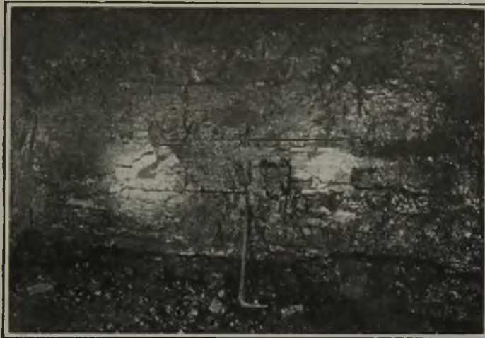
Fig. 6—Too Much Explosives Used in a Tight Shot
