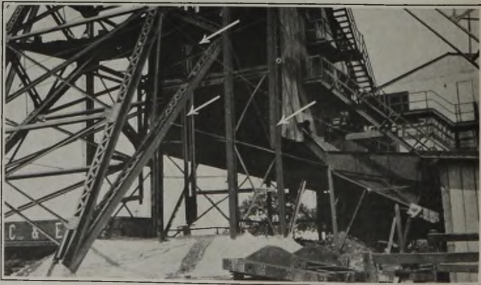
Ebbw Vale Coal Co.'s Shaft After Sealing Against Fire
