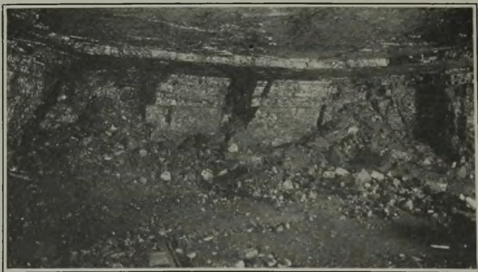
Blasted and Double-Sheared Room Face at Kathleen Mine
