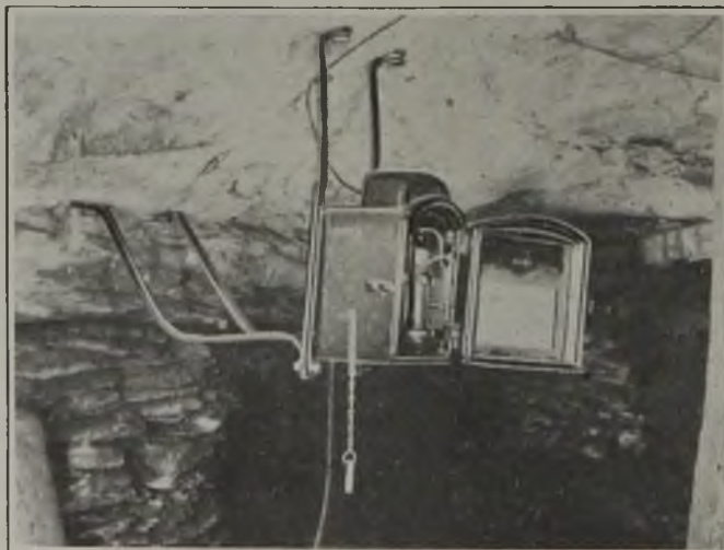
Telephone on Roof Bracket
