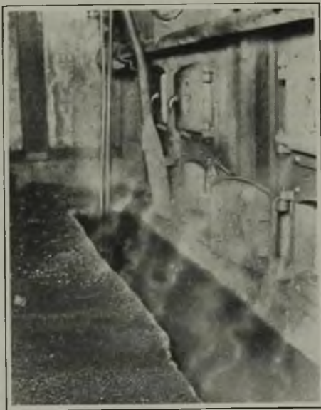
Trench in Front of Boilers
