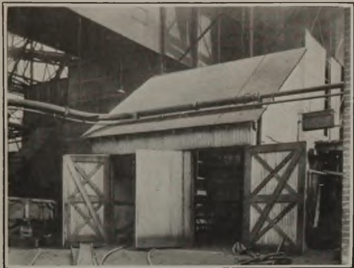
Fig. 1—Shelter in Which Air Is Pre-Heated
