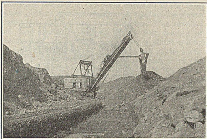
Dumping to the Spoil Bank
