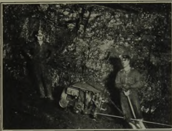
Shortwall Machine Cutting up Pitch in Gebo Mine
