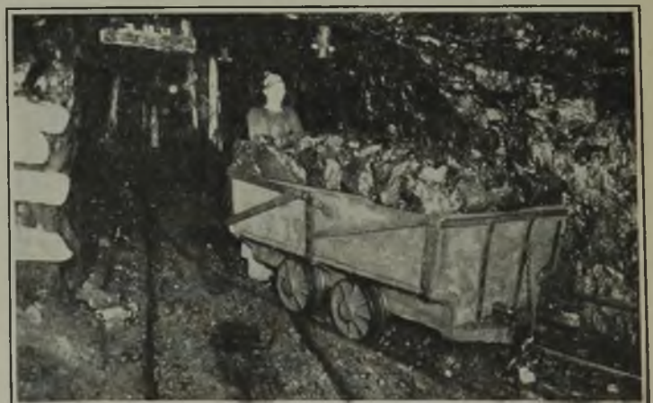
Gathering Hoist Pulls Car from Room, Gebo Mine
