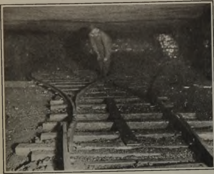
Fig. 3—Double Track to Facilitate Loading
