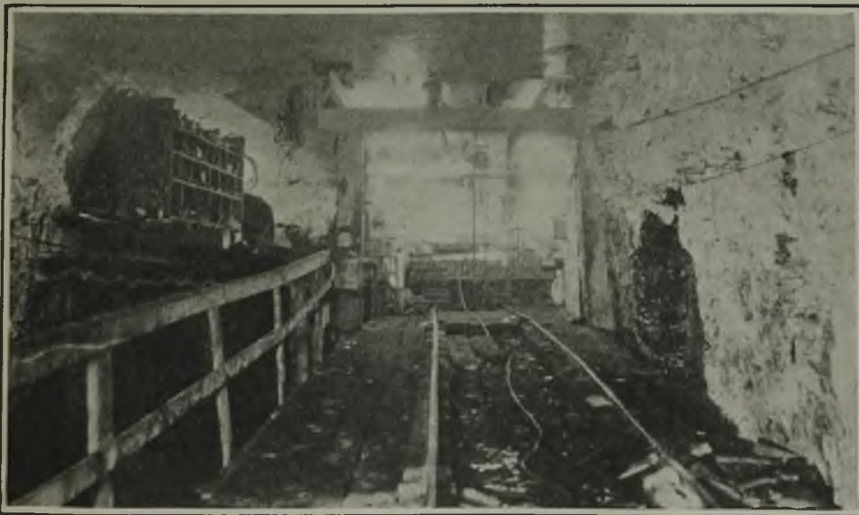
Underground Repair Shop with Good Drainage
