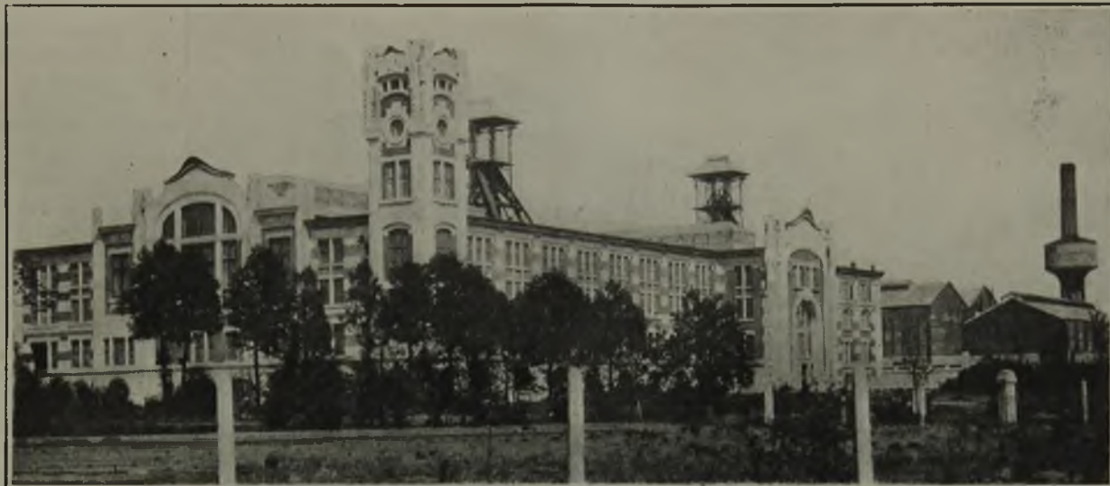
Office and Bathhouse at the André Dumont Colliery
