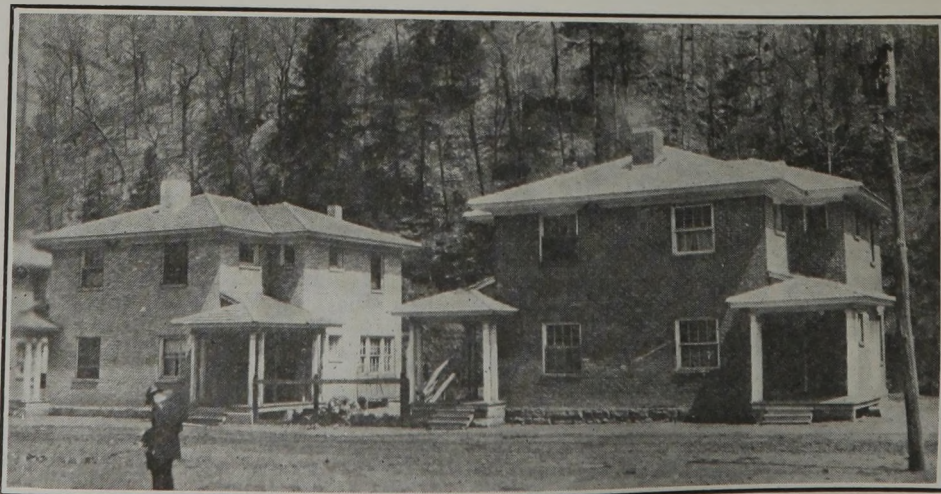
Substantial Dwellings Erected by the Kingston Pocahontas Coal Co.
