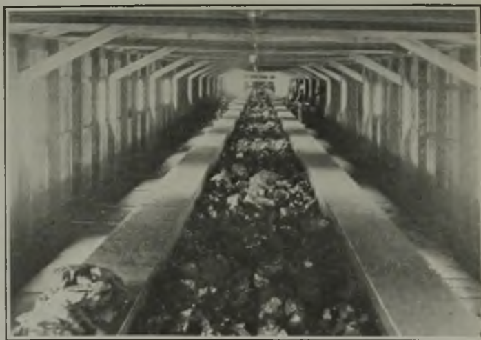
Fig. 4—One of the Horizontal Conveyors
