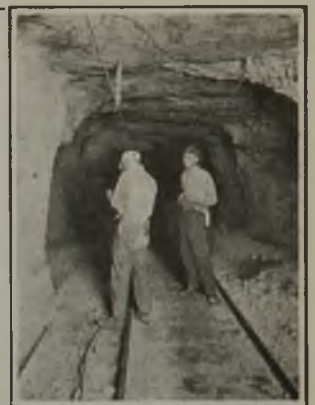
Mud-Sprayed Heading
