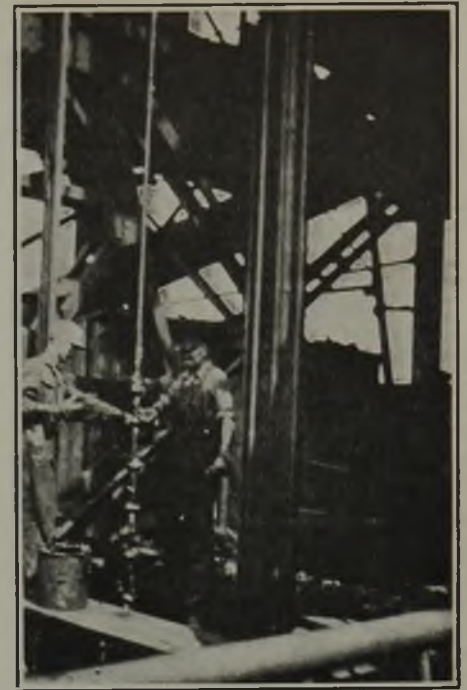
Greasing the Main Shaft Cable
