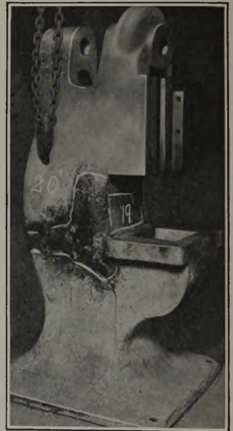
Fig. 1—Where First Fracture Occurred
