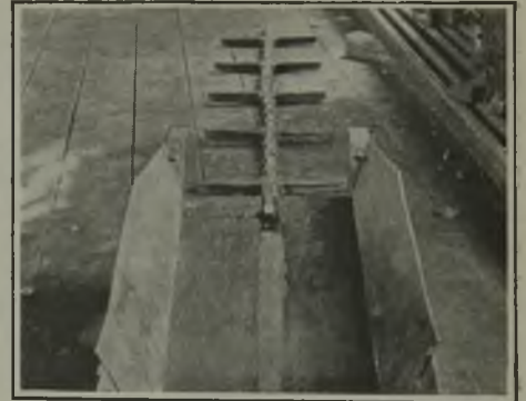
Fig. 3—Inserting a Conveyor Section
