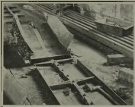
Fig. 1—Conveyor Tail Section Detached
