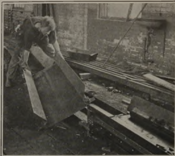
Fig. 6—Inserting a Straight Section
