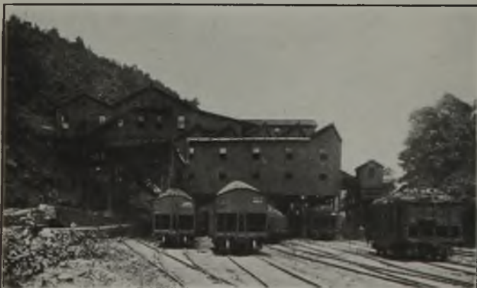
Tipple and Sizing Plant, Pocahontas Fuel Co.
