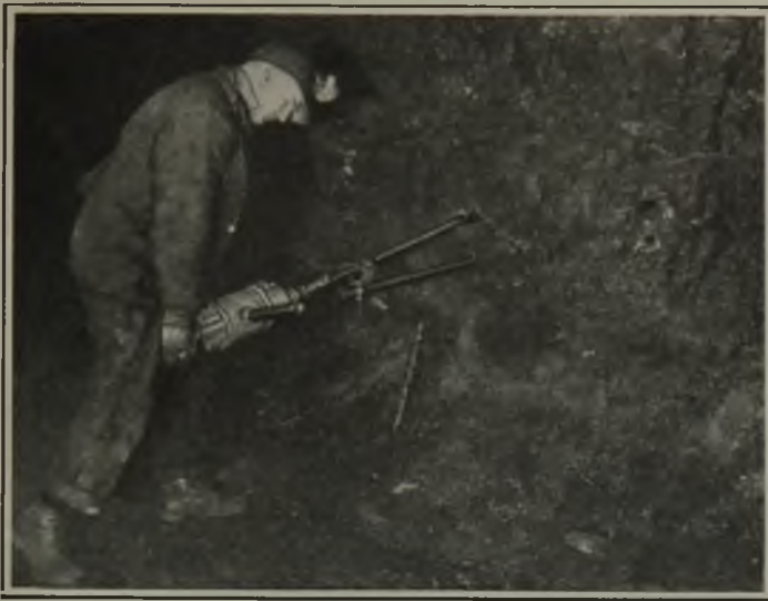
Drilling a Shot Hole Electrically
