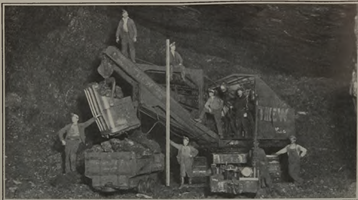
Thew Shovel in Hanna Mine
