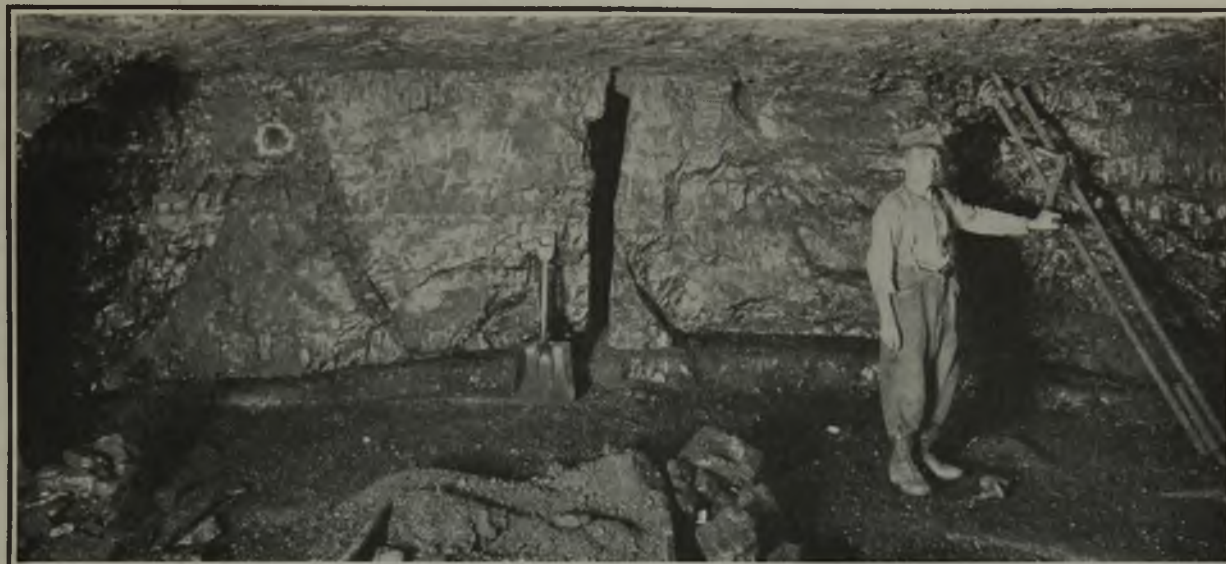
Drilling a Sheared Face
