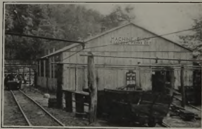
A Fabricated Shop in West Virginia
