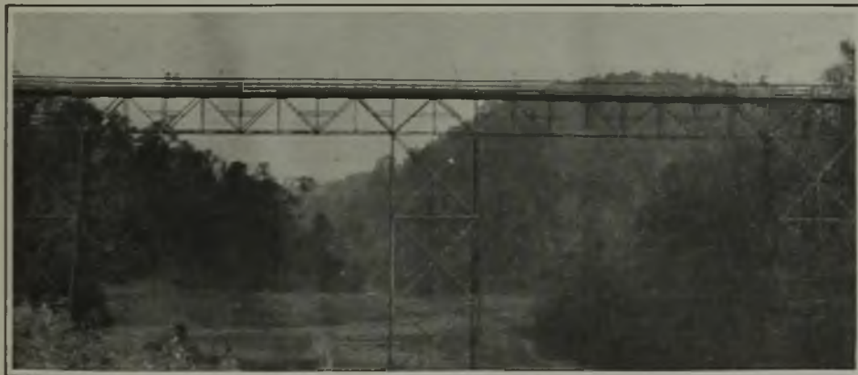
Main Haulage Road at No. 1 Mine North-East Coal Co.
