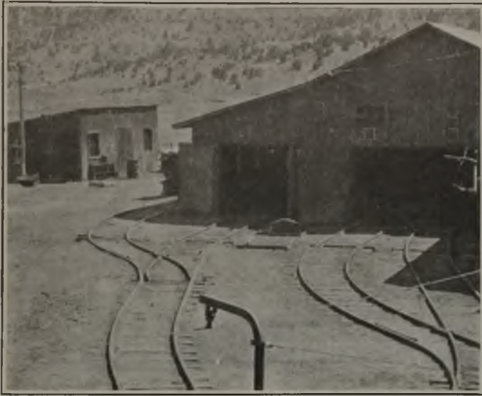
Fig. 6—A Clean Yard Bespeaks a Well-Ordered Mine
