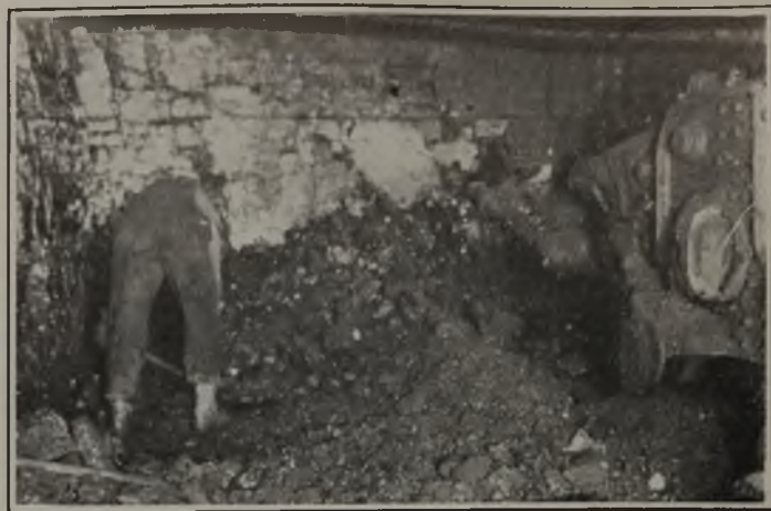
Fig. 2—Breaking Down a Hanging Shot
