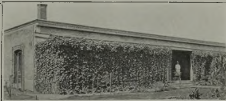
Manager's residence on right, a low ranging building with good ventilation and high rooms.
