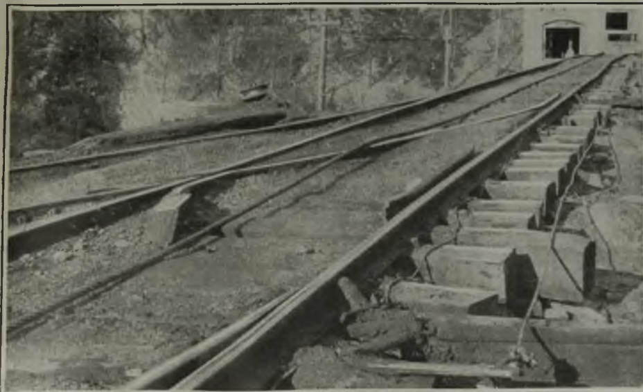
Fig. 1—Track Switch Operated from Hoist House
