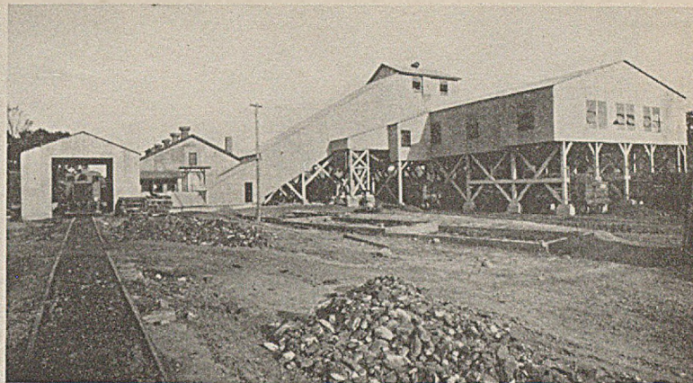
A Modern Stripping Tipple in Illinois
