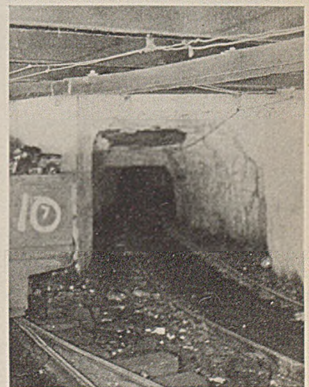
Belting Guards Trolley on Main Bottom
