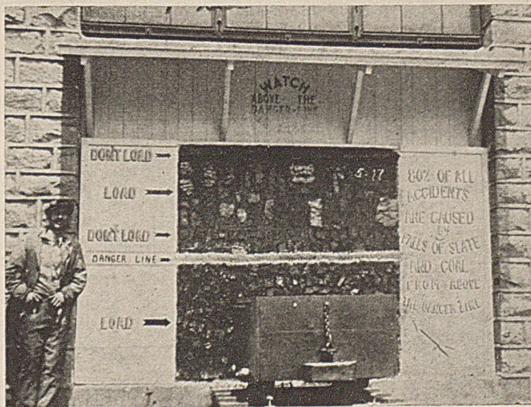
To Promote the Loading of Clean Coal and Doing It Safely
