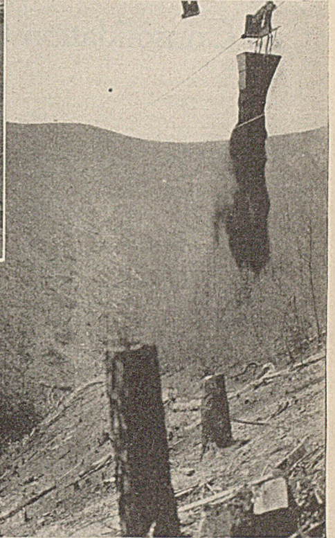
Dumping in 1,400-Ft. Span at Coalwood
