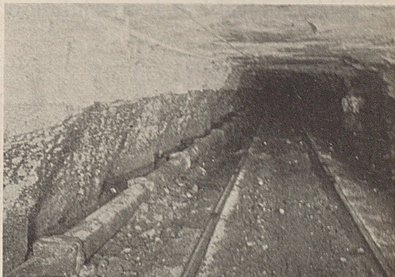
This Section of Line in Mine 120, Acosta, Pa., Contains 2,000 Ft. of 8-In. Cement-Lined Cast-Iron Pipe
