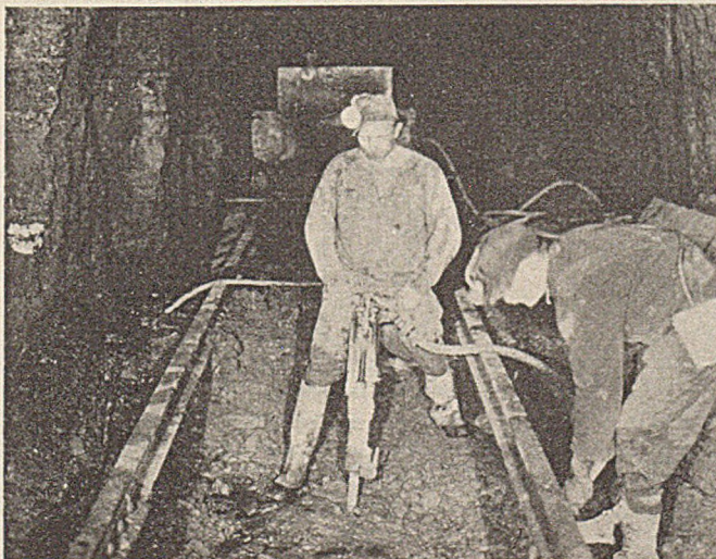
Fig. 2—One Man Loosens as Much Material as Four or Five Men With Picks
