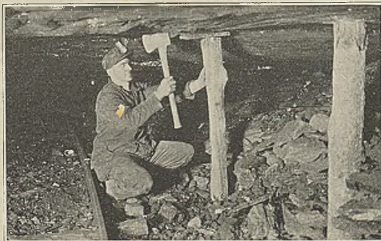
Fig. 15—Preparing to Hang Ventilating Tubing
