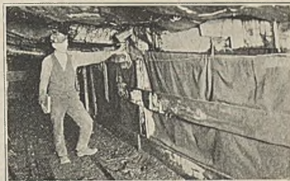
Fig. 13—Line Brattice at Side of Haulway
