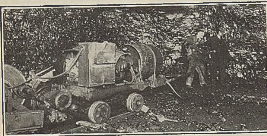
Drilling Shotholes by Machinery in 1926
