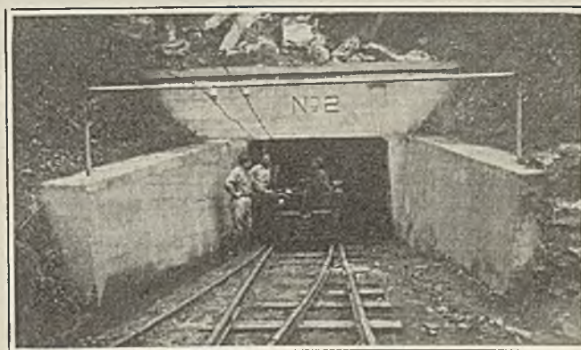
Haulage Locomotive Flagged at the Main Portal
