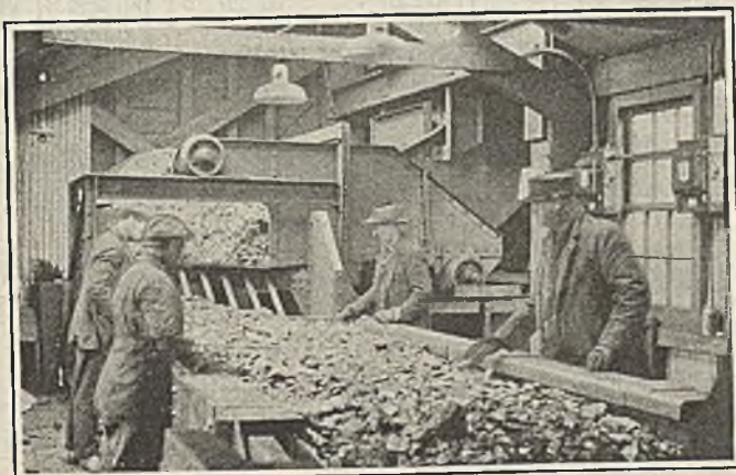
Good Light Aids Inspection
