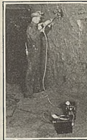
Cutting a Hitch in Coal Electrically
