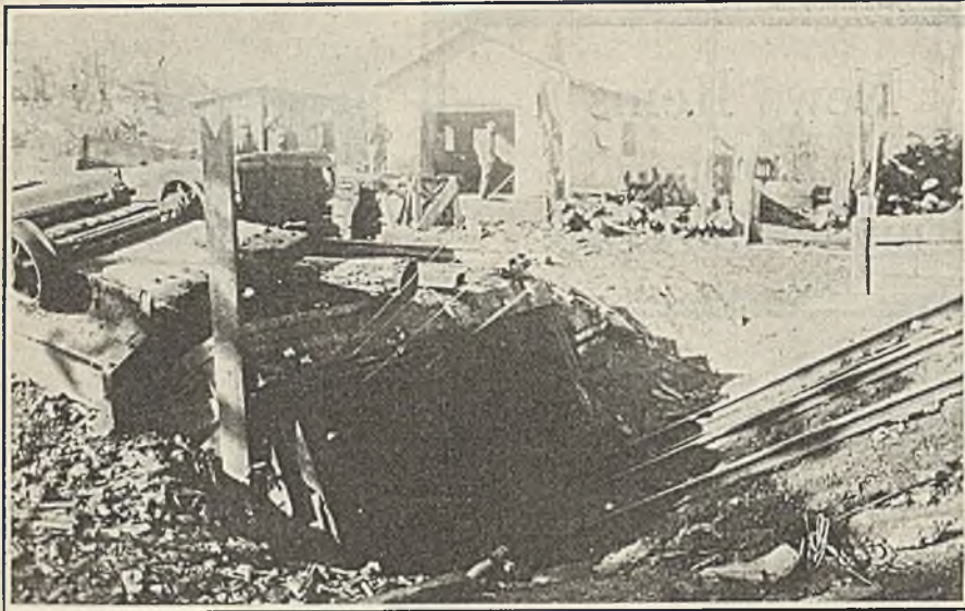
Portal of Main Slope, Mill Creek Coal Co.
