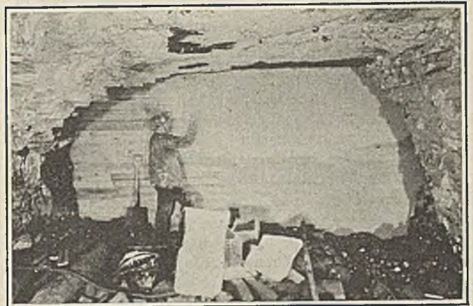
An Emergency Job Quickly Done
