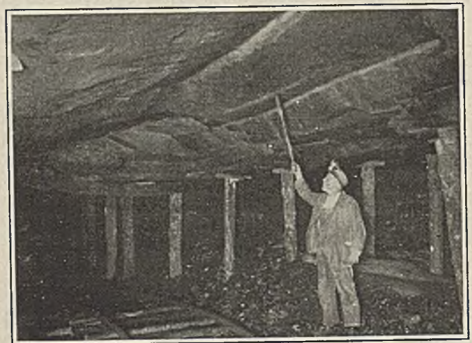
Fig. 2—A Horse-Back in Roof Along an Entry
