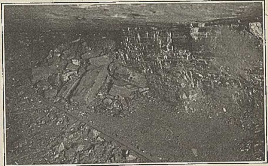
Coal Shot Down from First Cut of Room Neck
