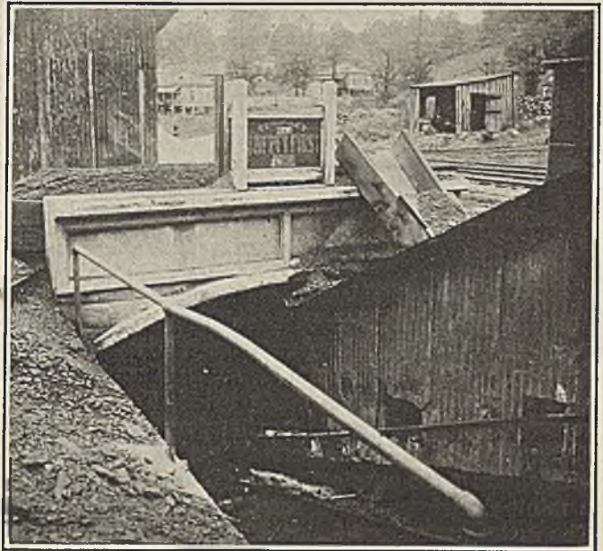
Portal of Slope Equipped with Belt Conveyor
