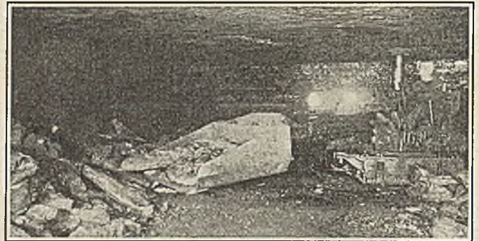
Gobbing the Heavy Parting Along the Left Rib
