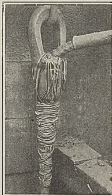
Close-Up of Cable Suspension
