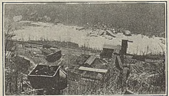
Looking Down Toward the New Tippel
