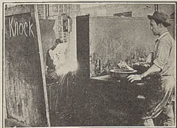
Shield Completely Encloses Arc Welder
