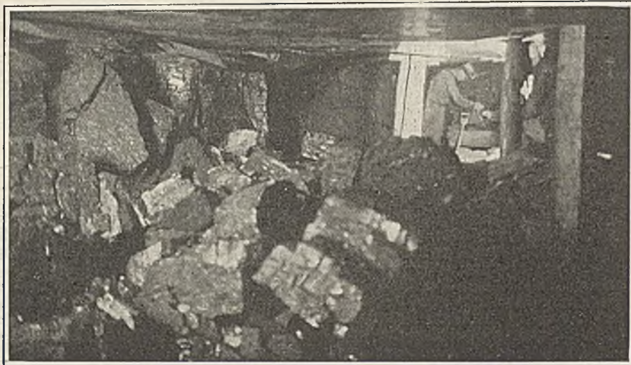
Loading in Room 35 Ft. Wide, High Splint Mine, Kentucky
