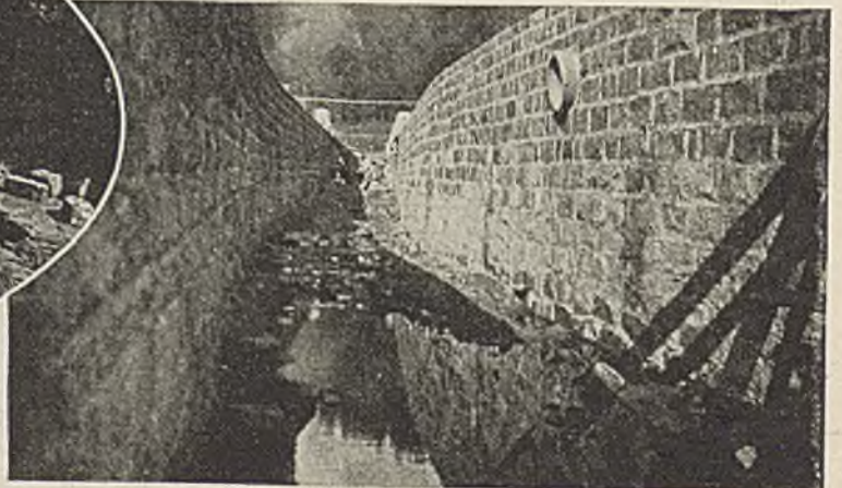
In the main creek culvert before the concrete top was applied.
