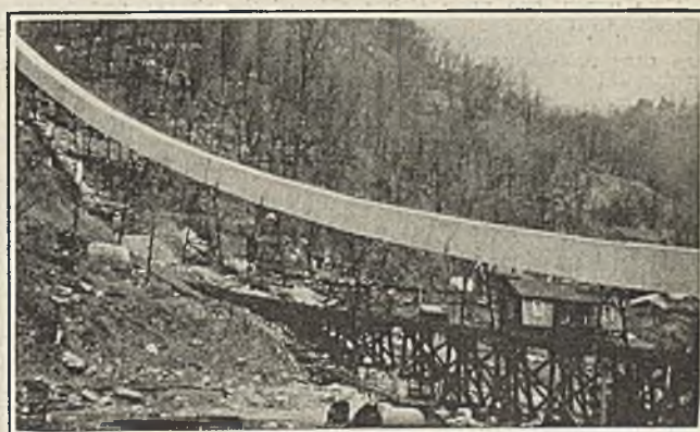
Lower End of Conveyor Gallery
