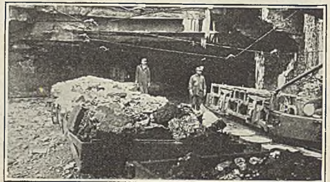
Mine Portal from Inside the Headhouse
