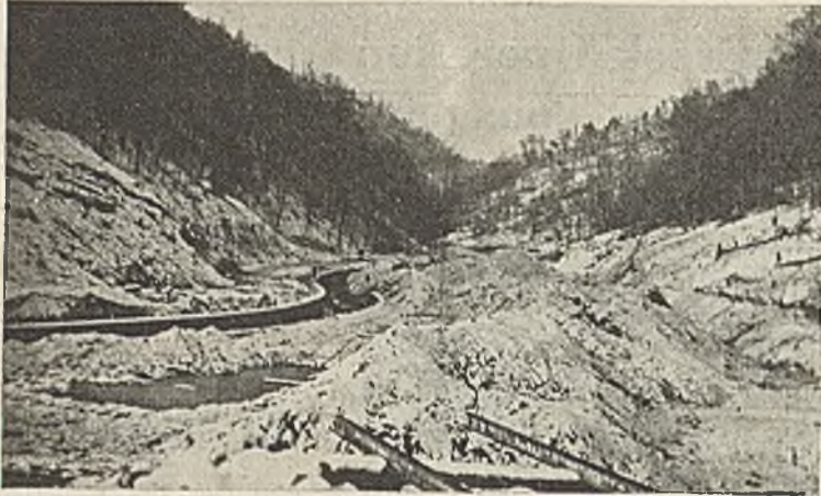
Winter view showing part of the town site. All of the building ground has to be "made." The creek is being confined to one side of the narrow valley or is being carried through large culverts, and the ground leveled the width of the valley for a distance of about 1½ miles. Space will be prepared for 200 double houses.
