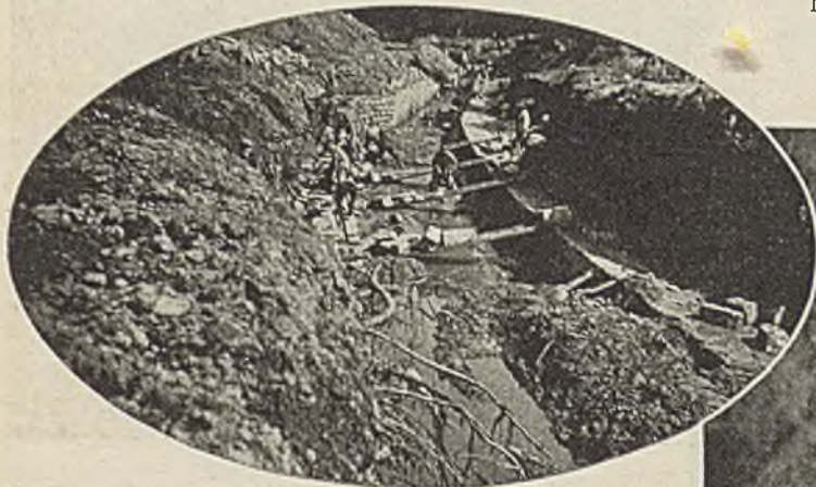
Working on the walls of the culvert.
