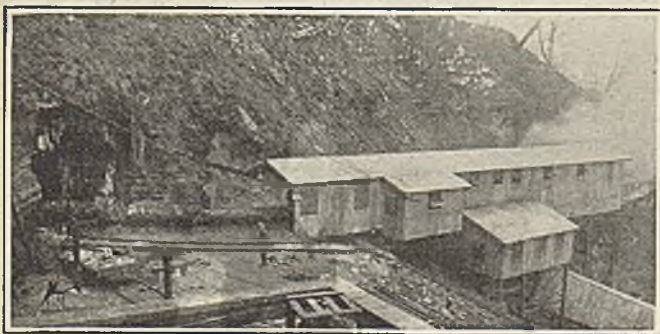
Recent View of the Completed Headhouse
