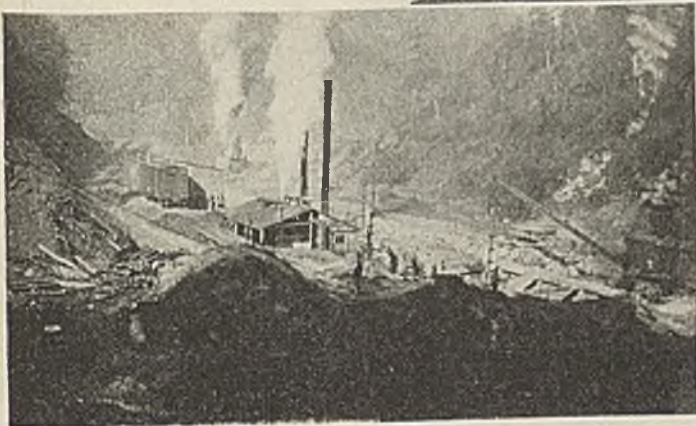
At right—Recent photograph of skip shaft. It is 11x32 ft., and like auxiliary shaft, will be concreted all the way down. Field mix being used is about 1-2.3-4. Three 2½-in. fiber conduits are being put into the wall of this shaft.
