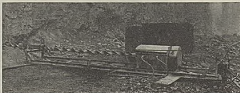
Fig. 2—Machine Drilling Horizontal Hole From Top of Coal Into High Wall at Allendale Mine.
