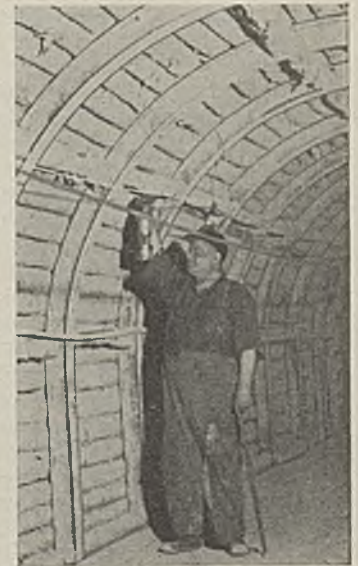
Fig. 1—Steel Timbers in a Nova Scotia Mine.
