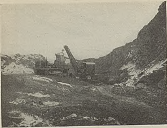
Fig. 3—Stripping the Orchard Bed, Kingston Colliery
