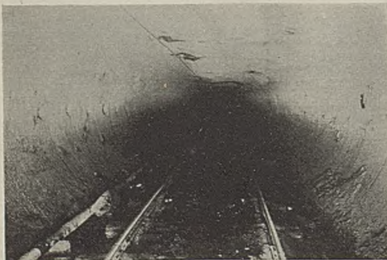
This Method Assures Straight, Smooth Ribs and Arches Which Generally Hold the Roof Secure Without Timbers.
