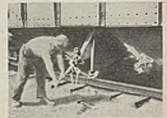
Prescott Safety Tool in Place for Closing Hopper Door
