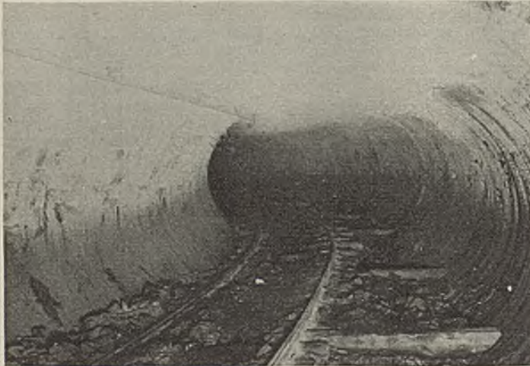
Curves Can Be Turned With the Entry Drivers With Almost as Much Facility and Smoothness as in the Advancing of Straightaways.
