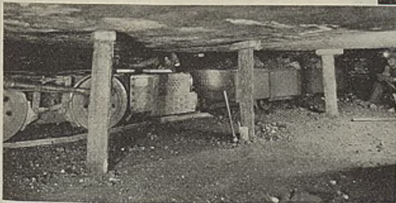
The Locomotive Has Arrived to Pull the Loaded Car From the Face and Replace It With an Empty.
