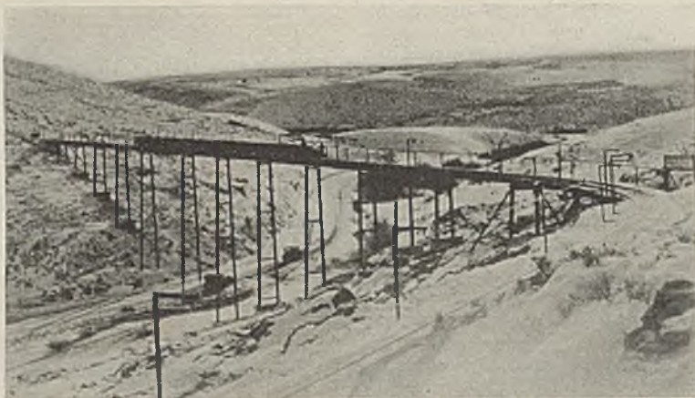
Pipe Bridge Built by the Kemmerer Coal Co. at Its New Opening
