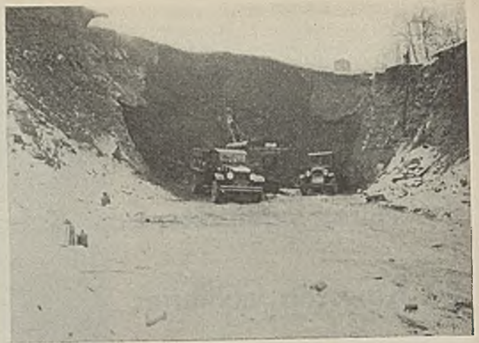
Fig. 4—Stripping Wash Over the Lance Vein, Kingston
