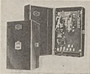
Cutler-Hammer Across-the-Line Starter
