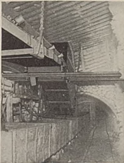
Fig. 8—Delivery End of Main Belt; Receiving Hopper and Trip Being Loaded.
