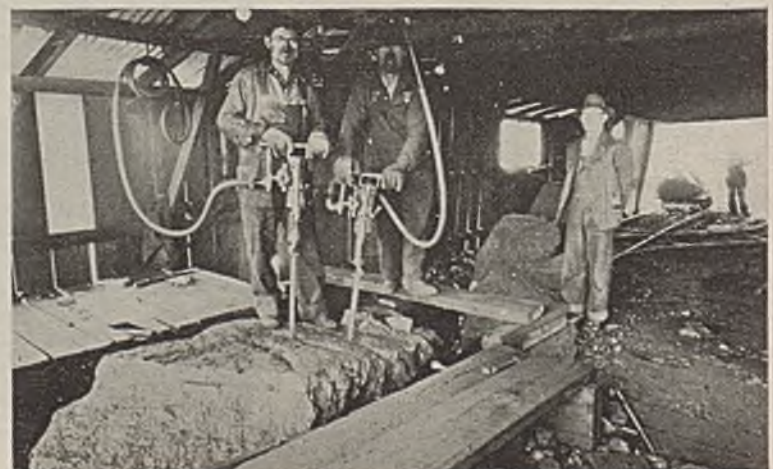
Fig. 5—Breaking a 3,800-Lb. Block to the Required Size
