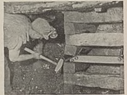
Fig. 3—Hardwood Chock With Releaser; Man About to Slip Catch
