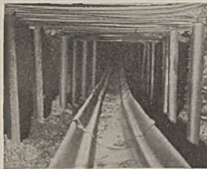
Fig. 1—Steel Props and Straps Protecting Face Conveyor
