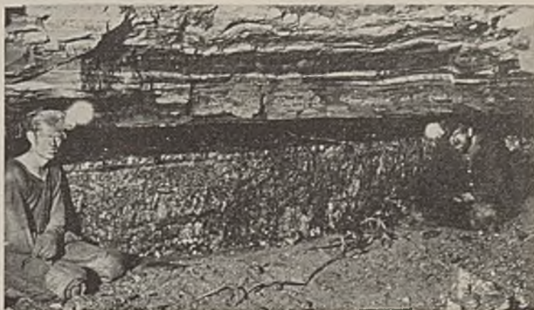
Fig. 1—Block at Road Head With Rope Around It Ready to Pull It on Mine Car
