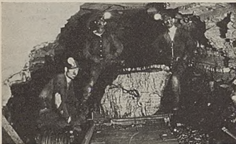
Fig. 3—Block of Coal Ready for Pulling on Mine Car; Winch Hoist on Left
