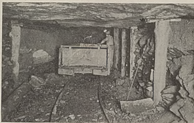
Fig. 3—Mining a Pillar After Flushing.
