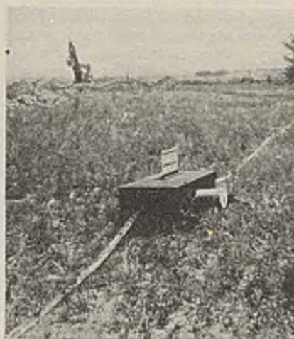
Junction Box Ready for Approaching Stripper to be Plugged In.
