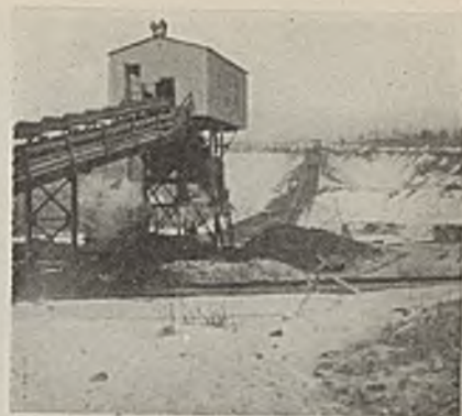
Refuse Loading Station and Incline
