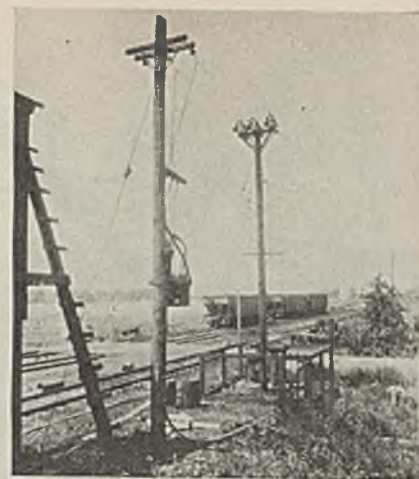
Junction of Pole Line and Ground Cable, Showing Lightning Arrestor and Oil Switch.
