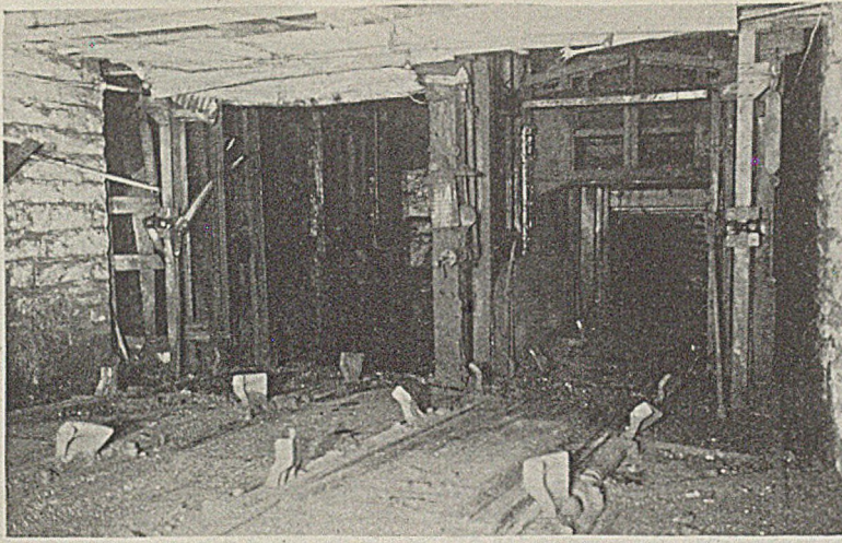
Caging Time Was Reduced by Installation of Horn Preopening Equipment
