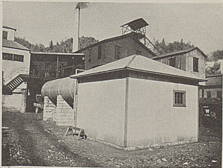
Storage Tank and Building in Foreground Handle and Mix Liquid Calcium Chloride
