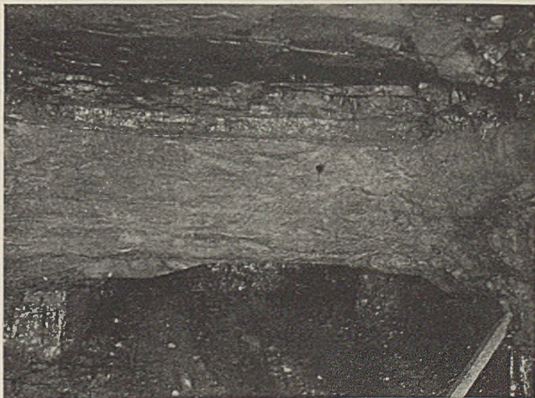
Fig. 1—Face of Haulage Heading With Coal Loaded but Before Top Rock Has Been Shot
