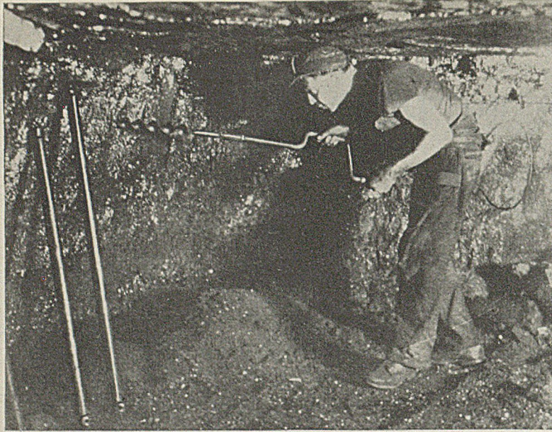
Drilling for Shell Blasting in No. 5 Mine
