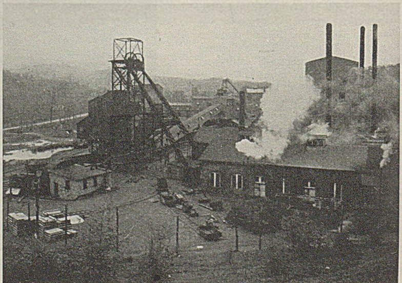
Surface Works at Nos. 5 and 6 Mines. Cleaning Plant Is on the Hill Behind the Boiler House. No. 6 Headframe Appears in the Background.
