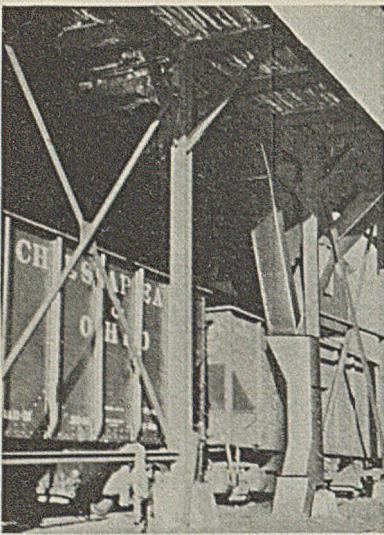
Fig. 3—Chutes Lead to an Underground Refuse Conveyor Which Runs at Right Angles to the Tracks
