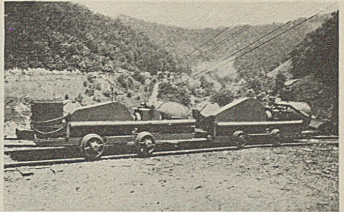
Portable Air Compressors After Overhauling and Installation of Automatic Starters and Drill Racks
