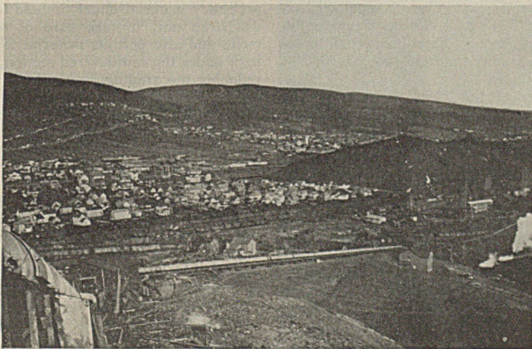
Fig. 3—Olyphant Disposal System; Old Bank Appears in the Background.
