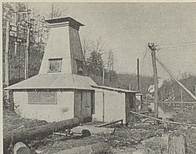
The Turbine Pump Housed in This Building Delivers Mine Water to the Pond for Boiler Feed. The Power Plant Is in the Background.
