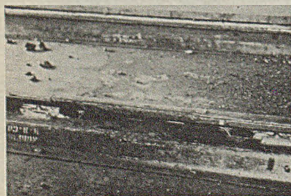
Showing Leaf-Spring Inserts in Top of Rail Above Printing Switches.
