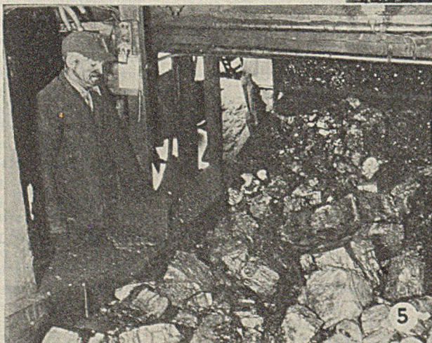
An Inspector Views the Coal From Each Car as It Passes by in a Thin Layer on an Apron Conveyor En Route Between the Dump and the Shaker Screens.
